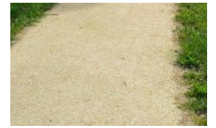
Halfverhard pad langs weg (Nobrecal o.g.)
